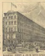
ROGERS, PEET & CO'S BUILDING.
